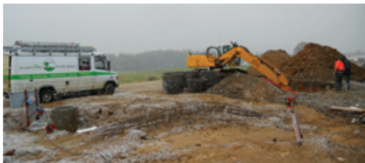
EnviTec is building two biogas plants in Latvia.
