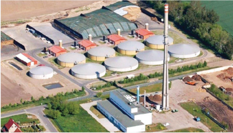
Plant produces just under 1.6 MW th per hour.
