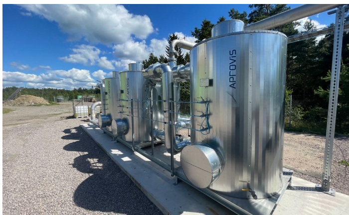
The skid-based raw gas upgrading system enables short installation times on site. (EnviTec Biogas AG)
