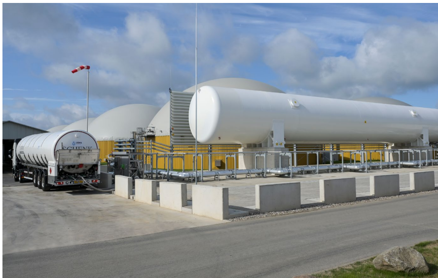
Up to 25,000 kg of bio-LNG per day and 18,000 tons of LCO 2 per year are produced here, primarily from agricultural residues. (EnviTec Biogas AG)
