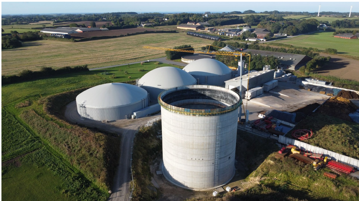
The 25-meter-high concrete fermenter was sunk seven meters deep into the ground. (EnviTec Biogas AG)
