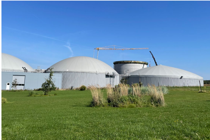
The industrial plant with attached EnviThan biogas upgrading system produces over 800 Nm 3 /h of high-purity biomethane and feeds it into the local gas grid. (EnviTec Biogas AG)
